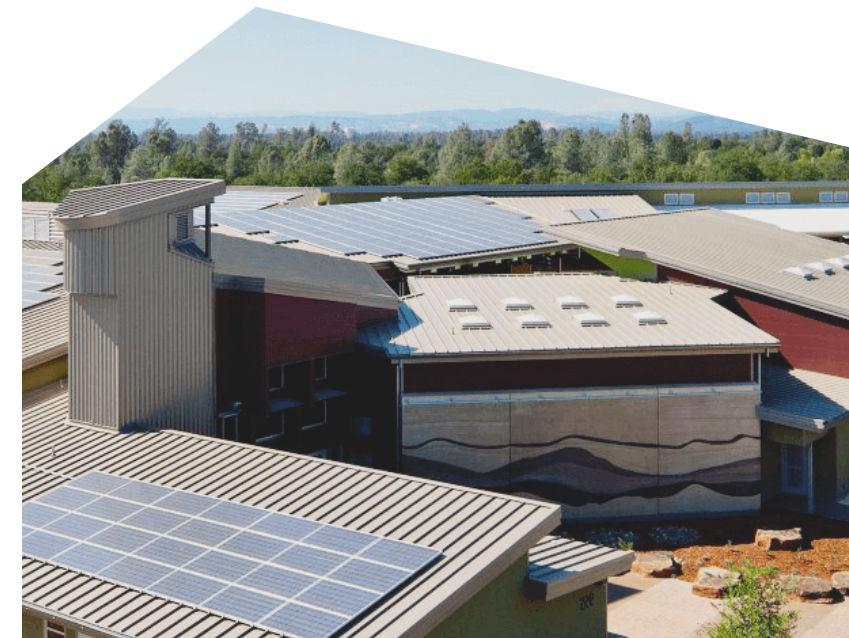
Metal cool roof at Redding School of the Arts. Photo courtesy of Kodiak Roofing.
