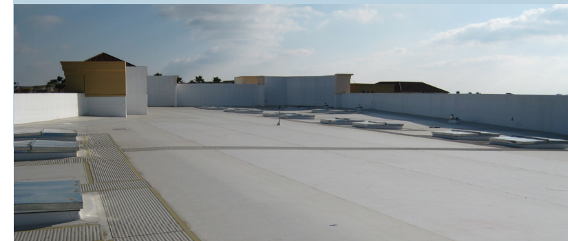
Cool roof coating at Palladio at Broadstone
