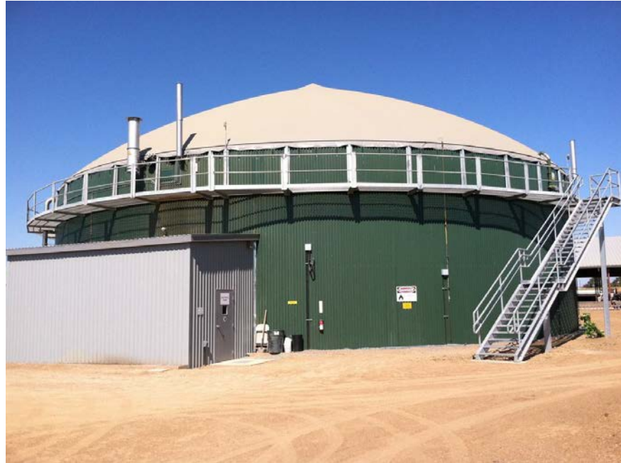
Figure 6: New Hope Tank Digester
