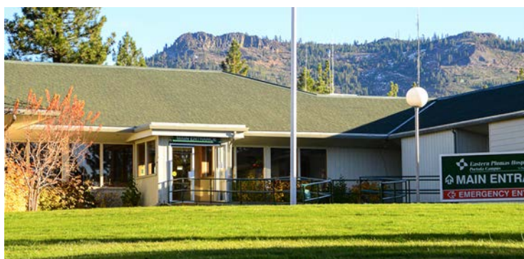
Figure 5: Eastern Plumas Health Care Site
