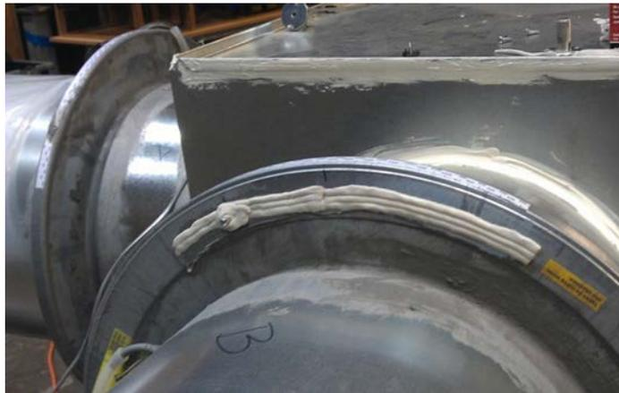
Mastic was used to seal duct seams and rope caulking used to seal branch iris damper control slot.
